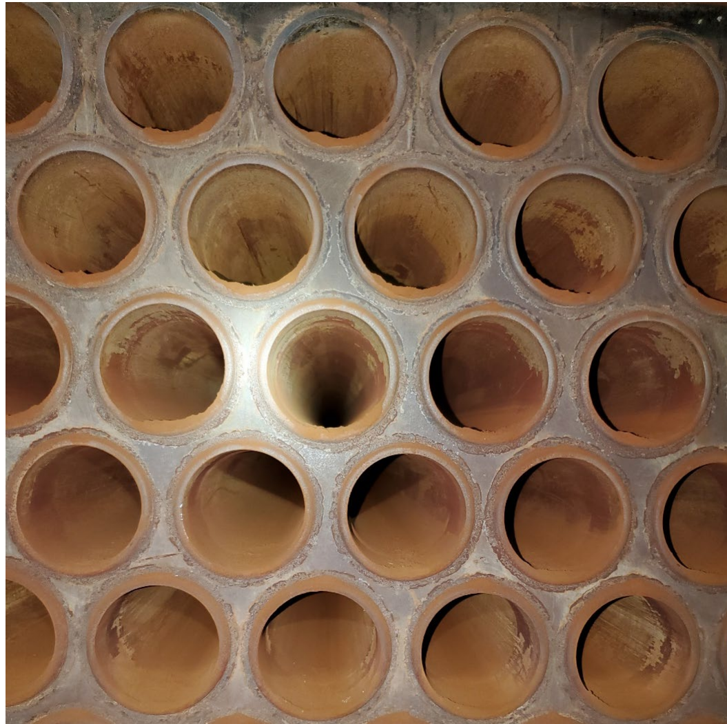
Visual inspection of boiler firetubes
