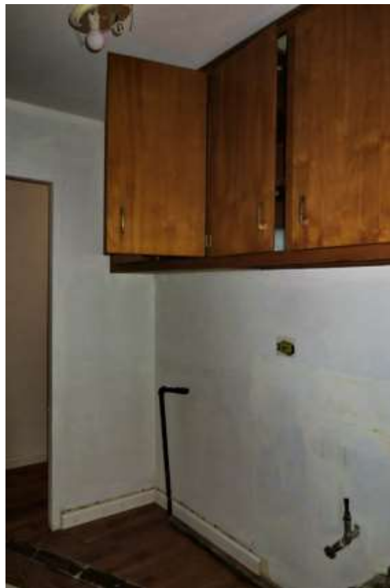
Apartment renovation for turnover.
