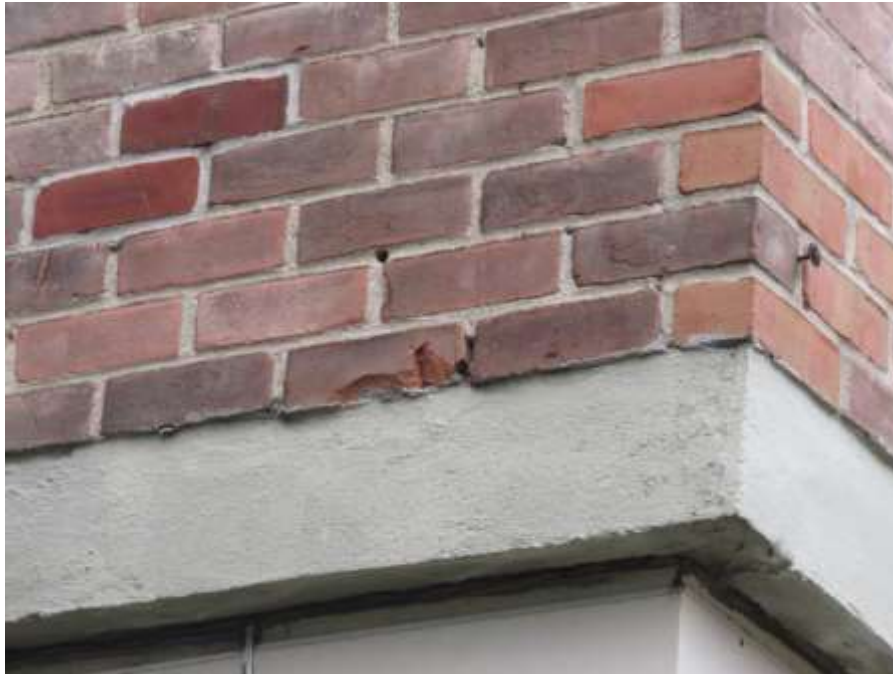
Spalled brick
