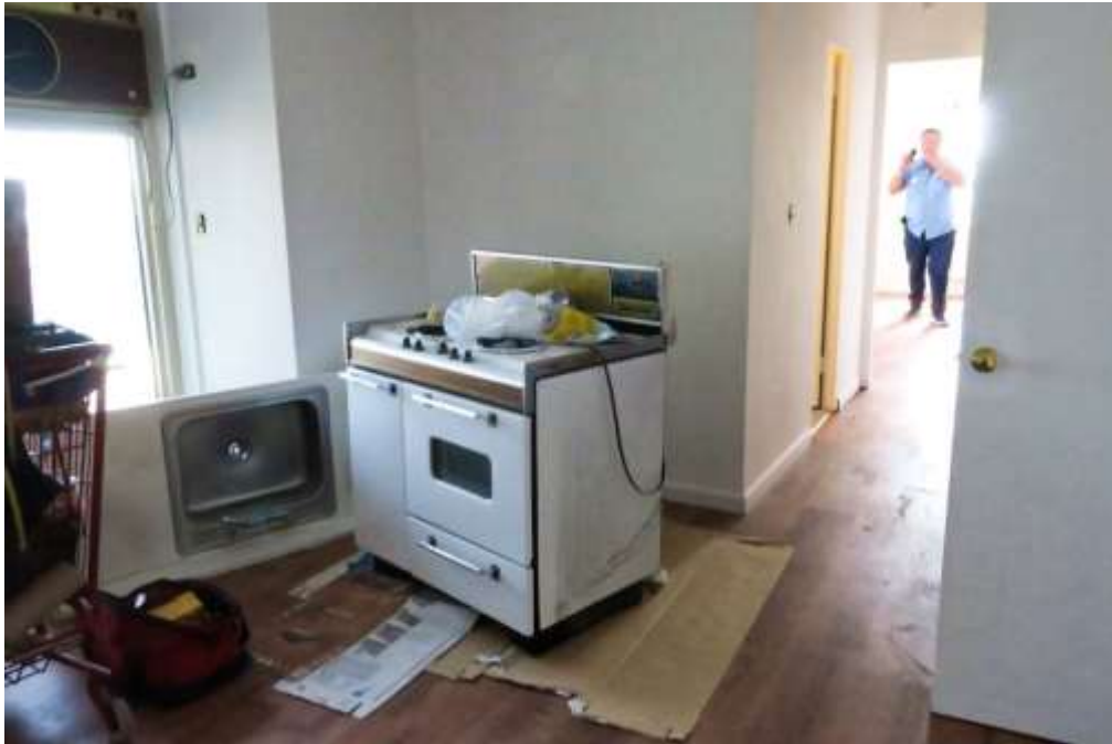
Apartment renovation for turnover.
