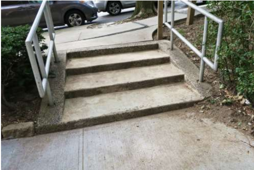
Typical exterior stair with railing
