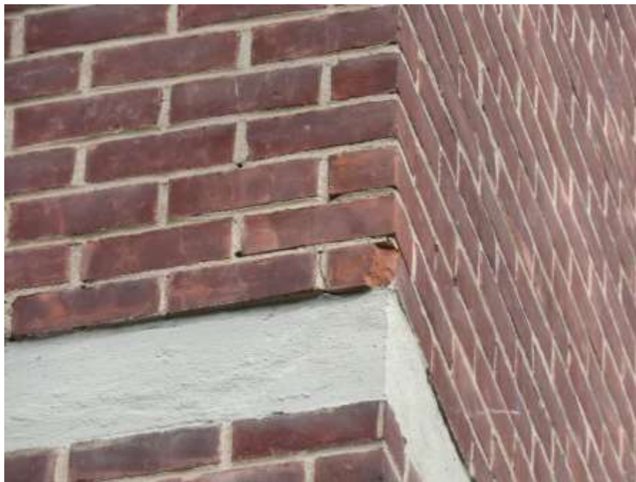
Spalled brick
