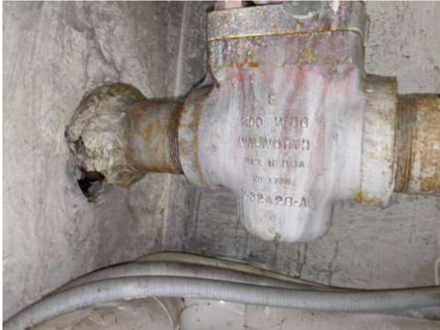
Typical Gas Service Shut-off Valve
