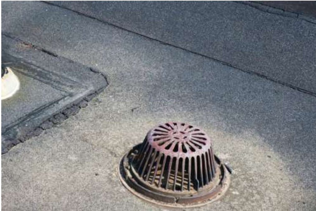
Typical roof drain
