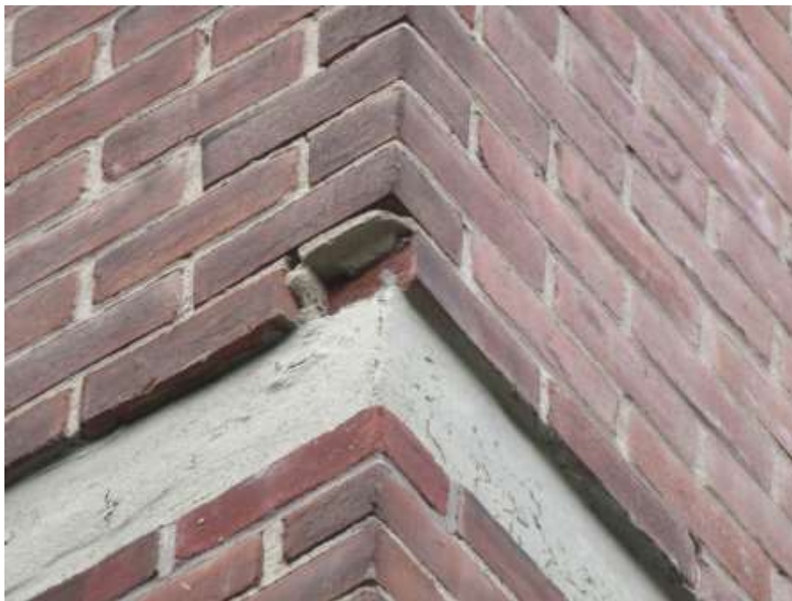
Spalled brick
