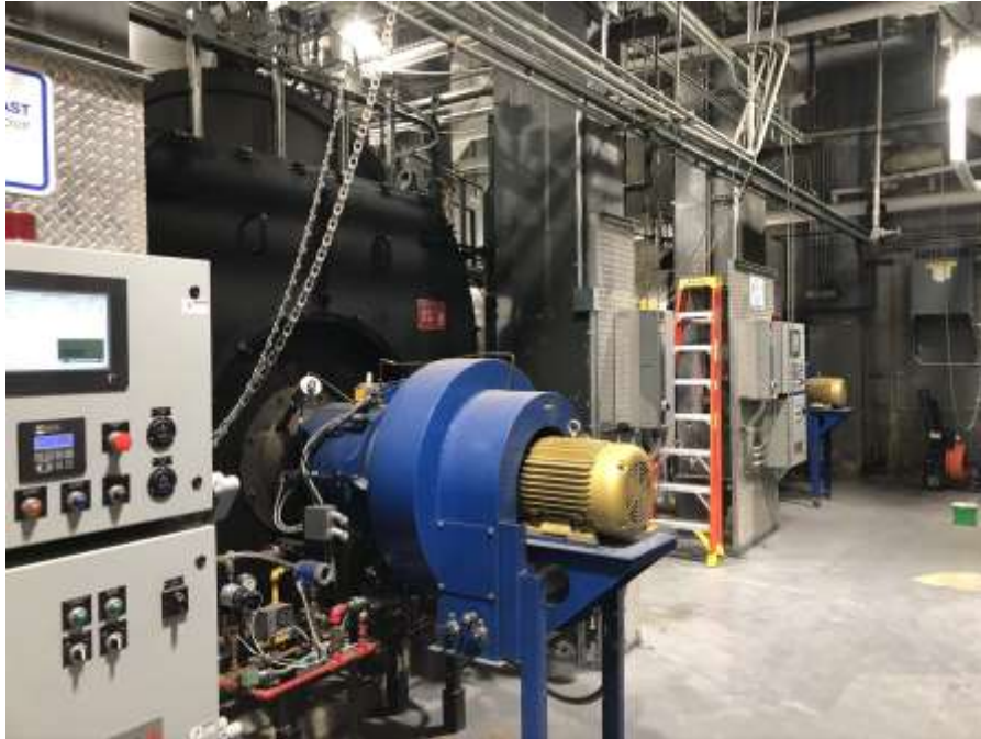
Typical Boiler and Burner
