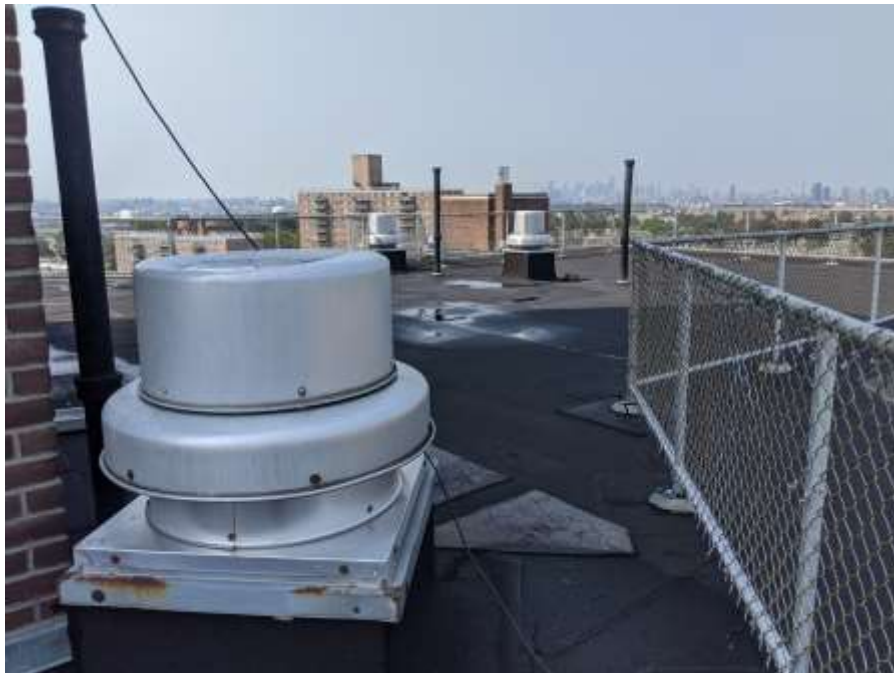
Typical Roof Exhaust Fan Upgraded – Roof
