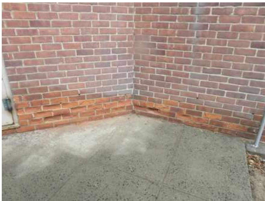
Spalled bricks
