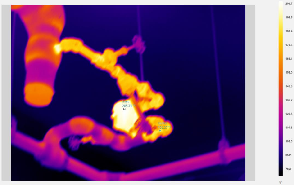
Building 2 Basement Trap A
