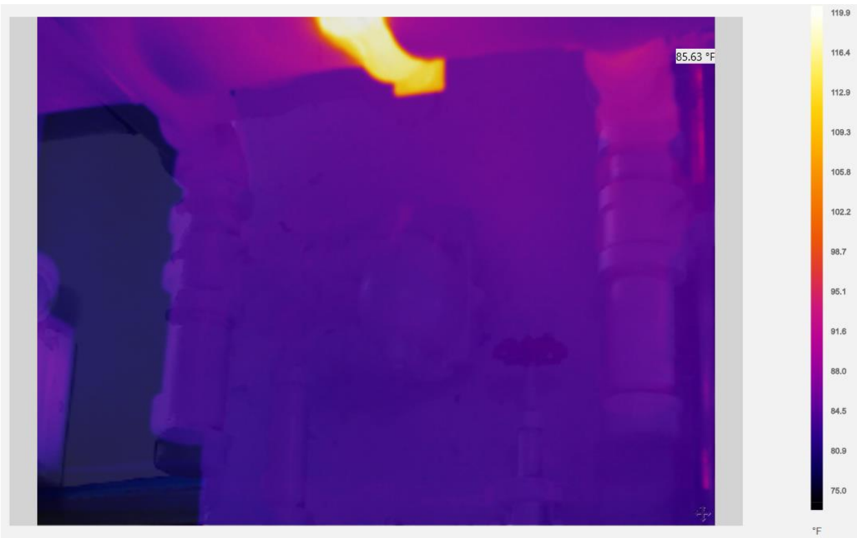
Building 3 Basement Trap B (not active)
