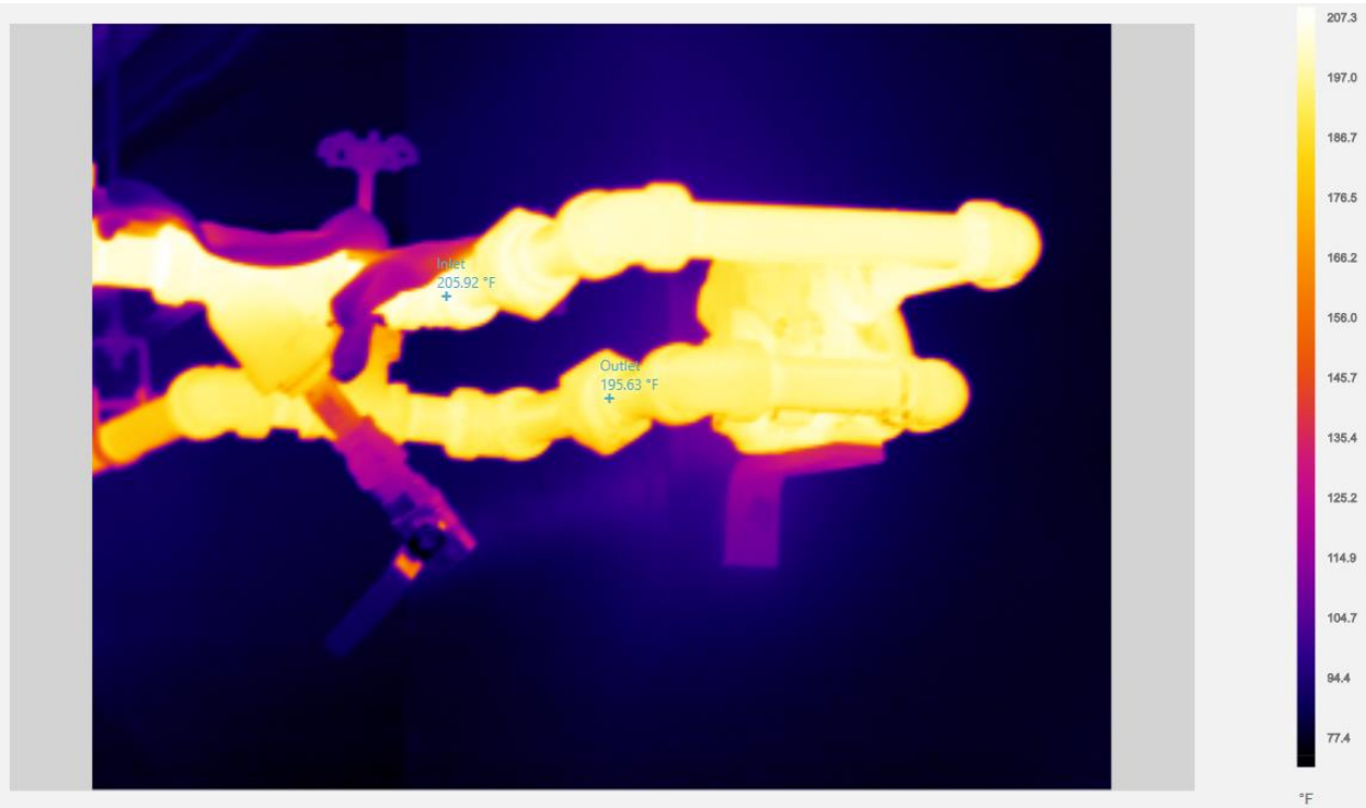
Building 7 Basement Trap B
